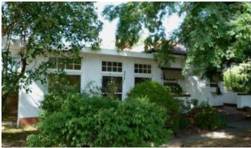
39 Bridge Street West, Benalla
